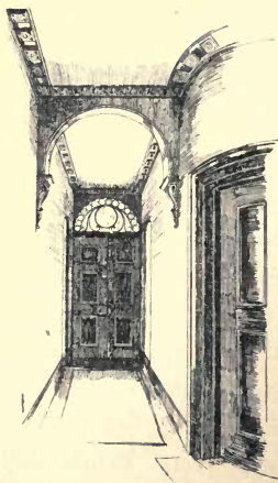
Entrance Hall of House at No. 13 Great Coram Street.
